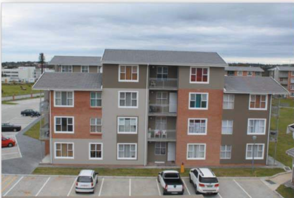
FAIRVIEW LINK, PORT ELIZABETH
